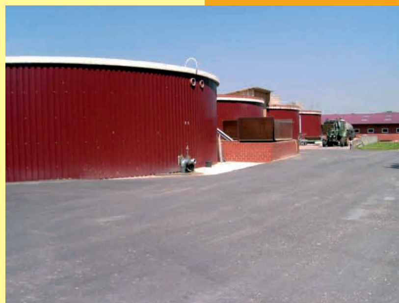
Biogasanlage in Bosse
